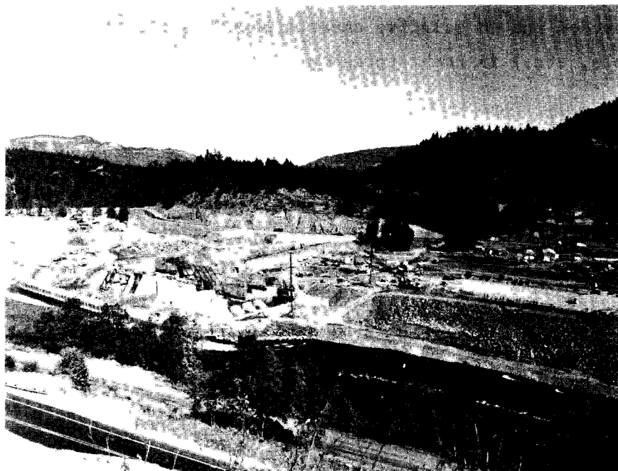
Cole M. Rivers Fish Hatchery, under construction
