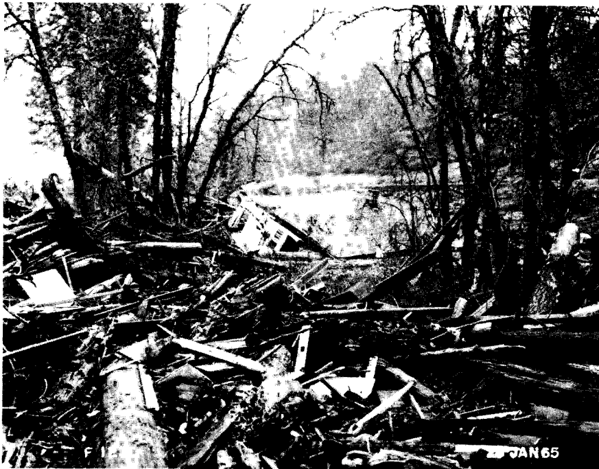
Flood Damage along Rogue River
